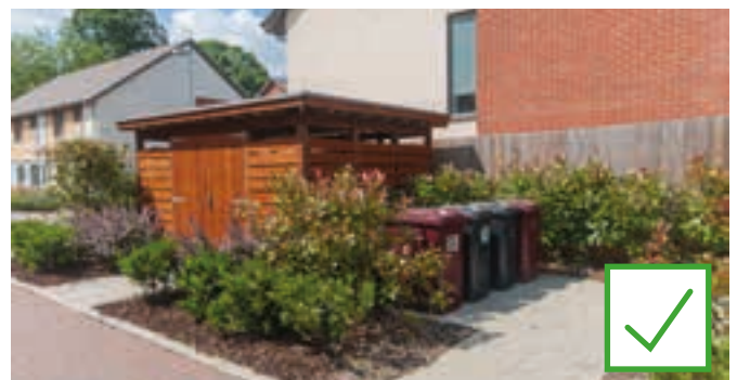
Communal bin / bike stores for apartment blocks must be sited unobtrusively, and should not dominate the street frontage.
