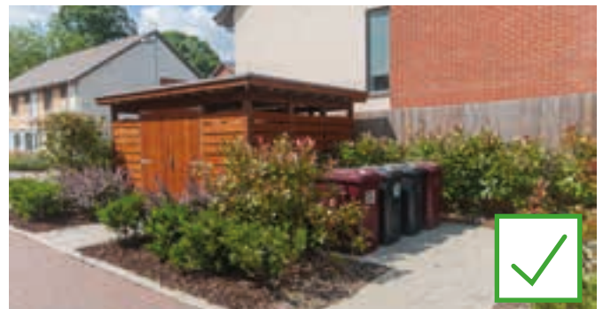
Communal bin / bike stores for apartment blocks must be sited unobtrusively, and should not dominate the street frontage.
