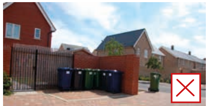
Open bins at main entrance of dwellings / apartment block are not acceptable.
